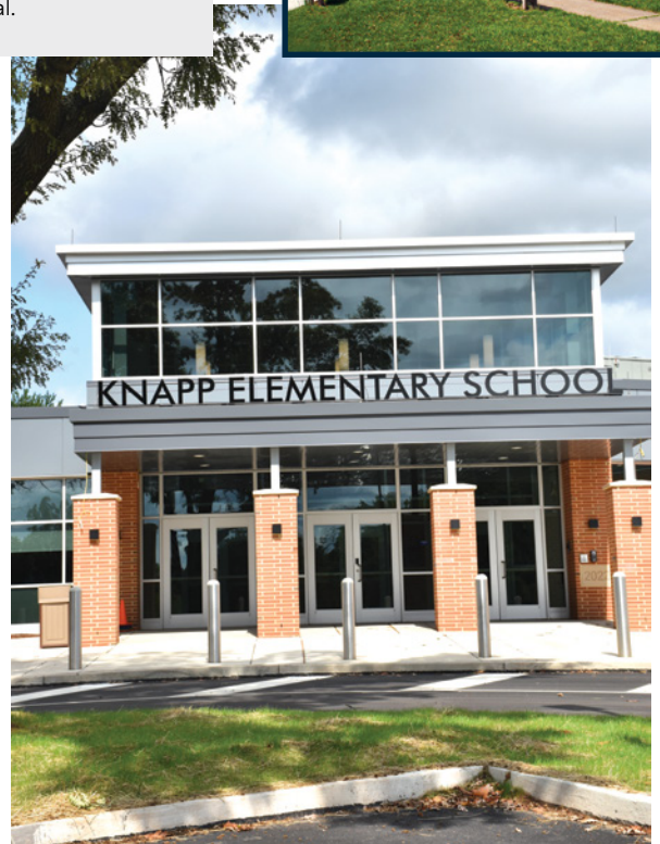
BEFORE (TOP RIGHT) AND AFTER (RIGHT) PHOTOS SHOWCASE THE TRANSFORMATION AT KNAPP ELEMENTARY SCHOOL FROM THE START OF THE PROJECT IN 2020 TO COMPLETION IN 2022.
